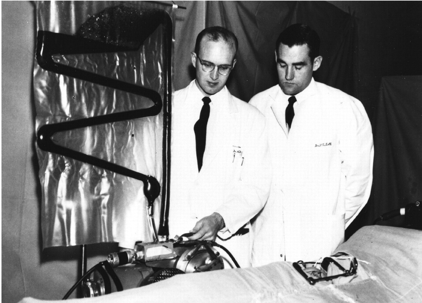
Richard DeWall and Vincent Gott standing beside a Travenol disposable bubble oxygenator.
